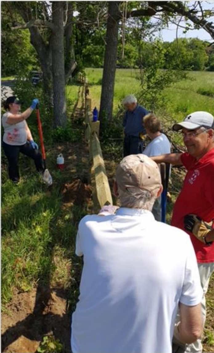
Larry Yost (back to camera) sighting the fence line (R. Bilsback photo)
