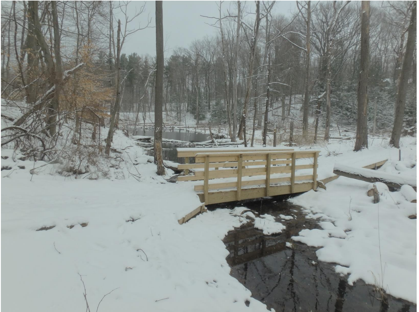
New Bridge from Big Field to Big Woods at GBWNP
