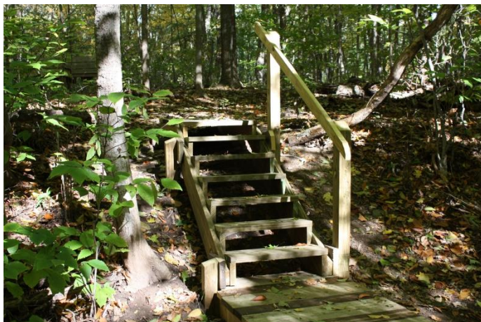
New Stairs at FMCP (D. Kuhn photo)
