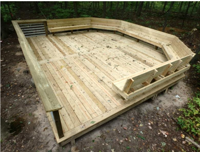
New Platform at Hickory Bark
