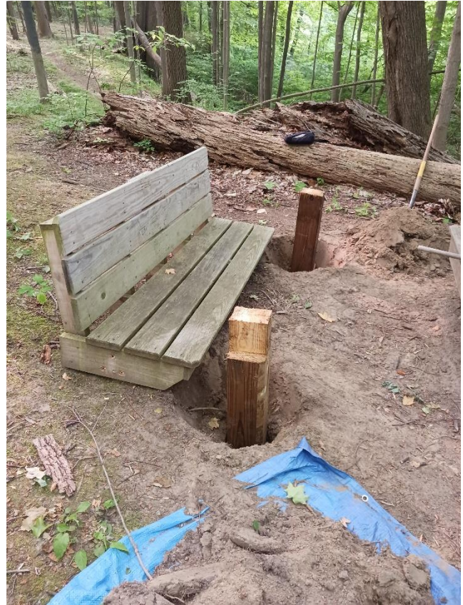
JUNT Bench repair in progress
